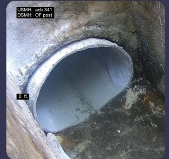
After Concrete Lining
