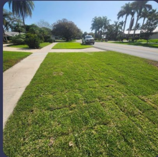
After Swale Renovation
