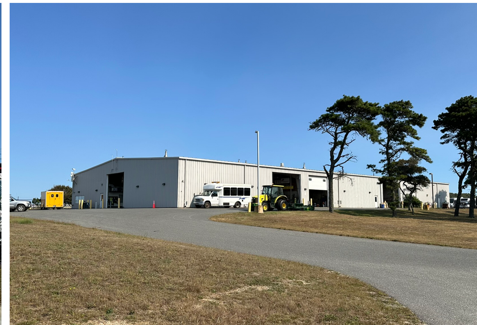
NANTUCKET AIRPORT 39 BUNKER RD FLEET STORAGE AND MAINTENANCE GARAGE FOR NANTUCKET MEMORIAL AIRPORT. SIMILAR ROOF LINES, METAL BUILDING, METAL ROOF.
