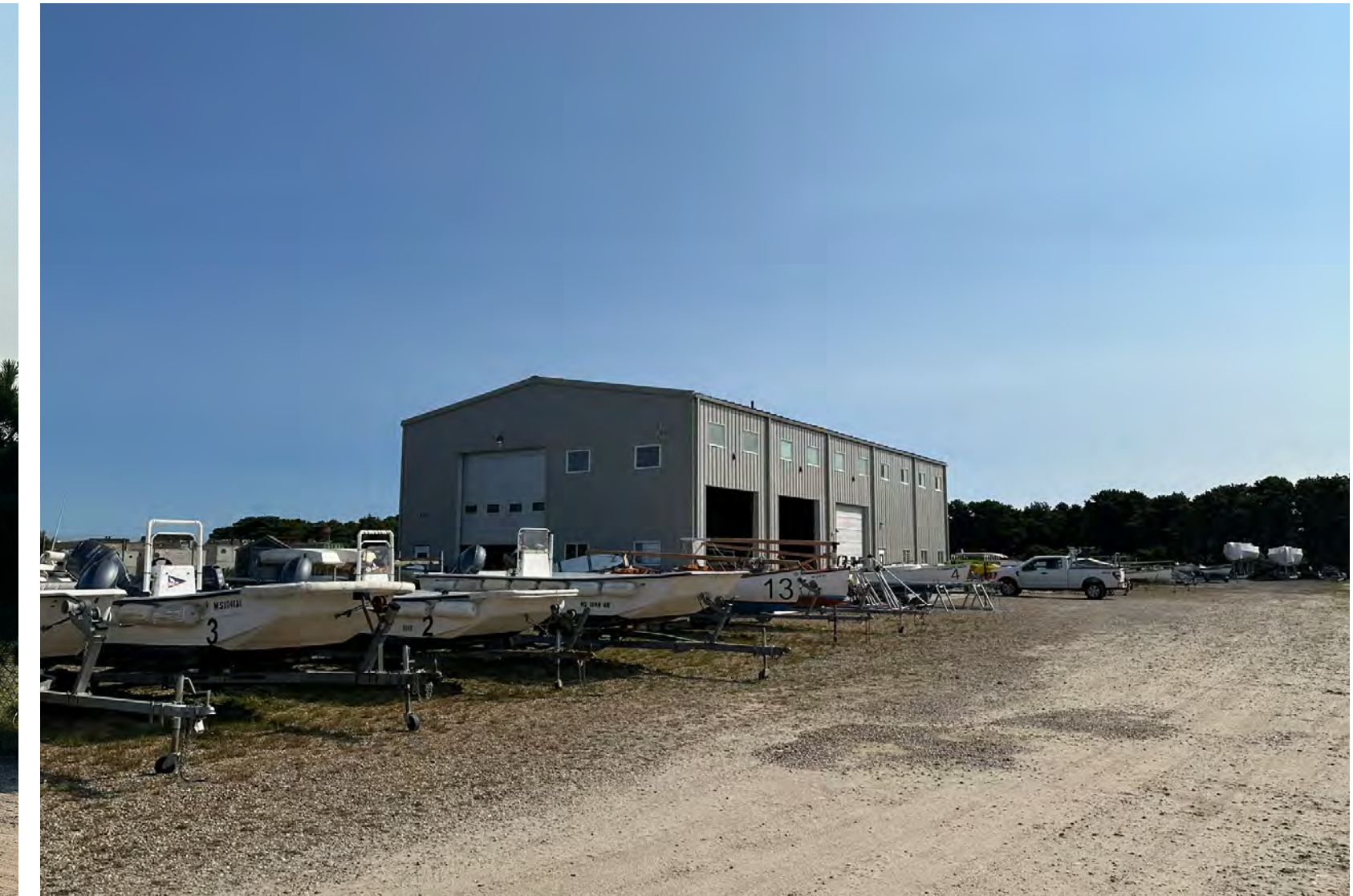
TON - COMMUNITY SAILING 12 INDUSTRY RD TALL METAL BUILDING WITH METAL ROOF; SIMILAR HEIGHT AT OVERHEAD DOORS TO WHAT IS PROPOSED AT DPW BUILDING.
