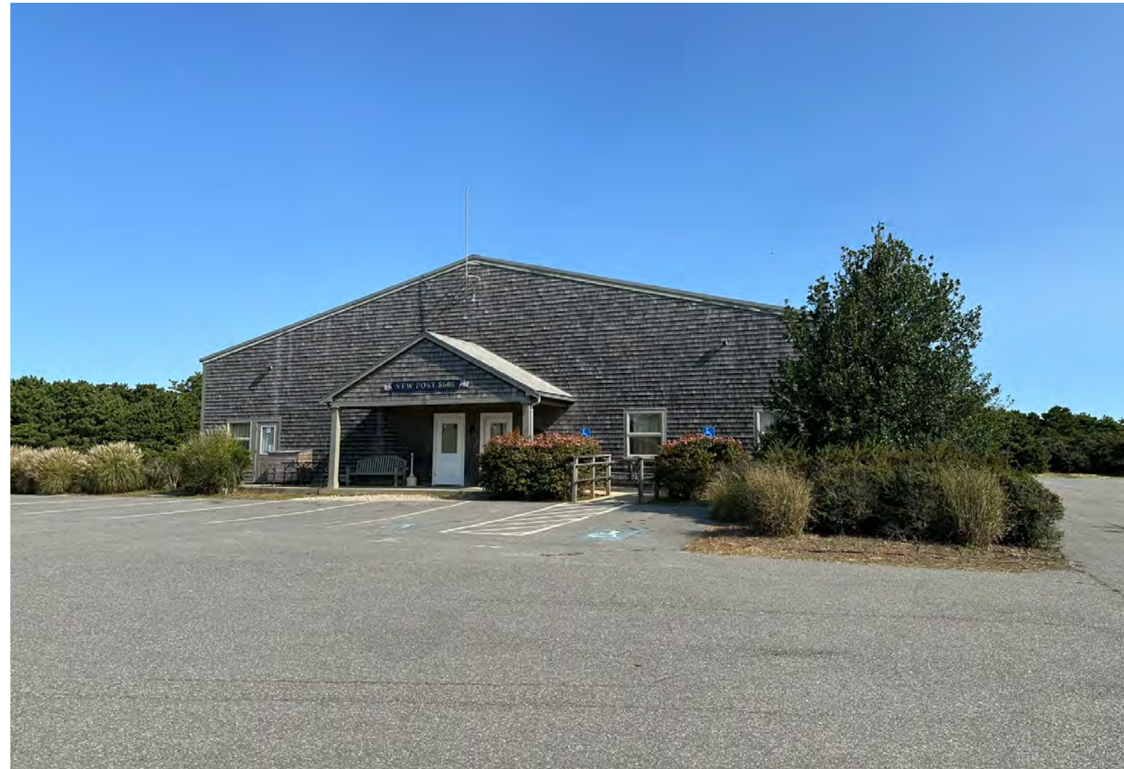
VFW BUILDING 22 BUNKER RD FIRST BUILDING DRIVEN BY ON THE WAY TO THE DPW.
