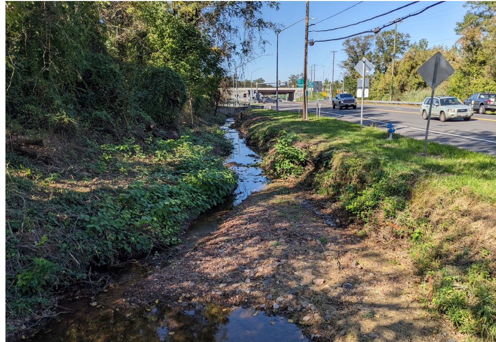
Highland Drive culvert, looking downstream.
