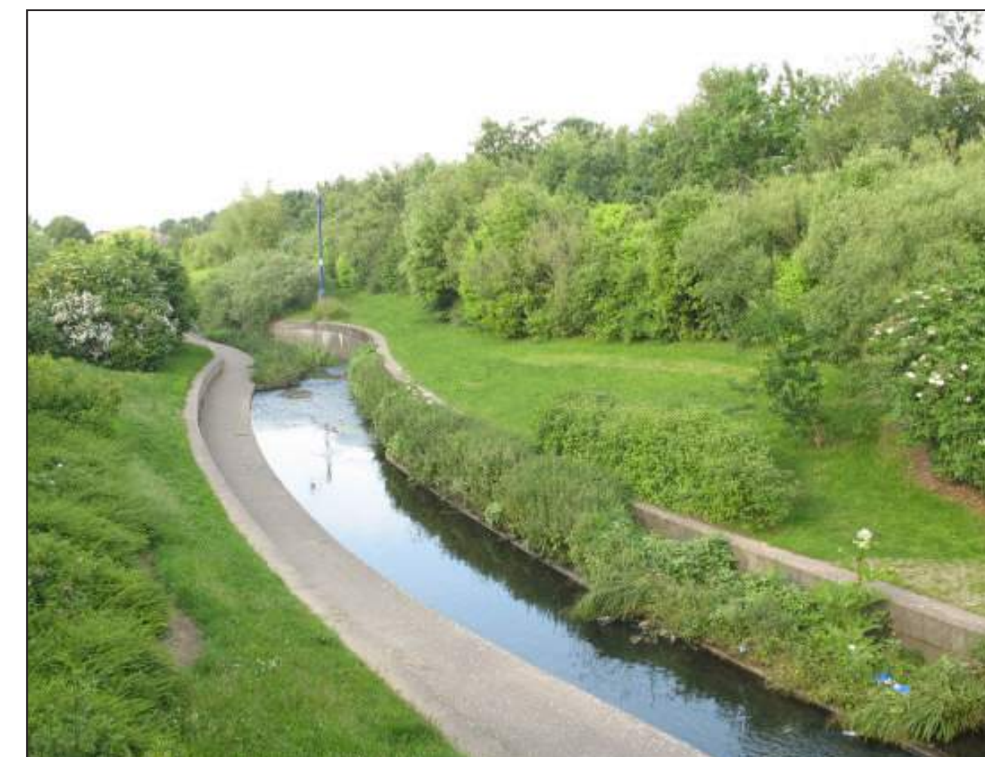
Connecting the river Ravensbourne to Catford
