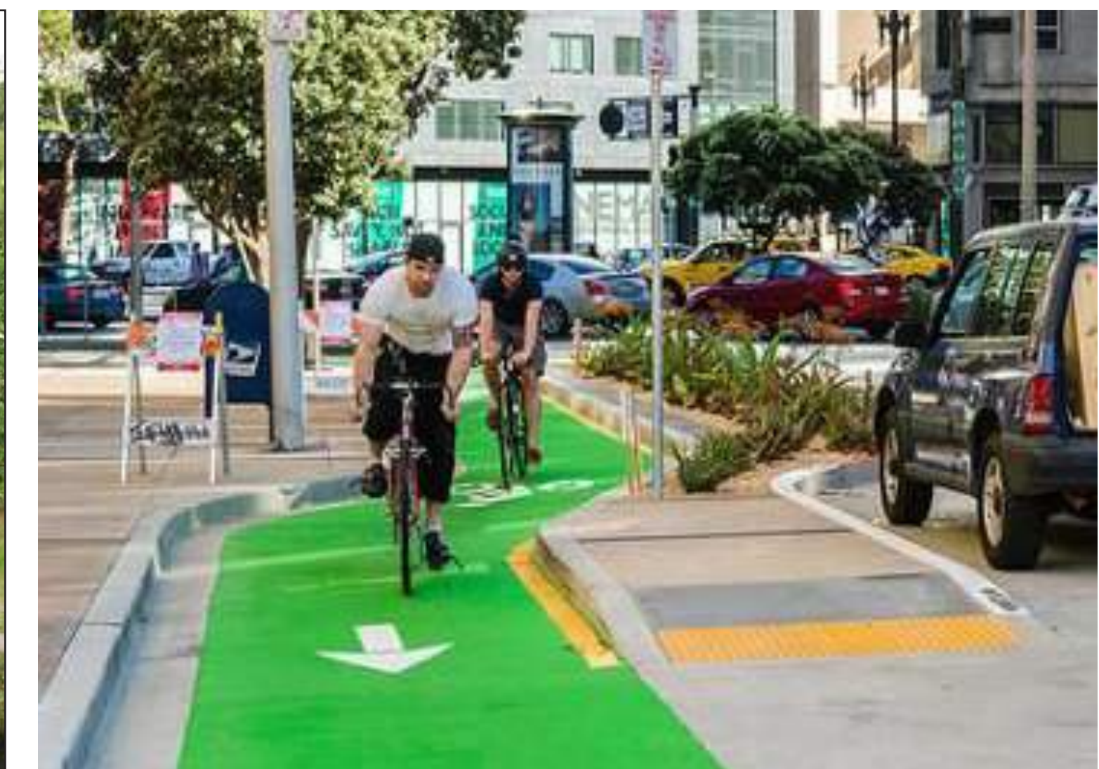
Clearly demarcated cycle tracks
