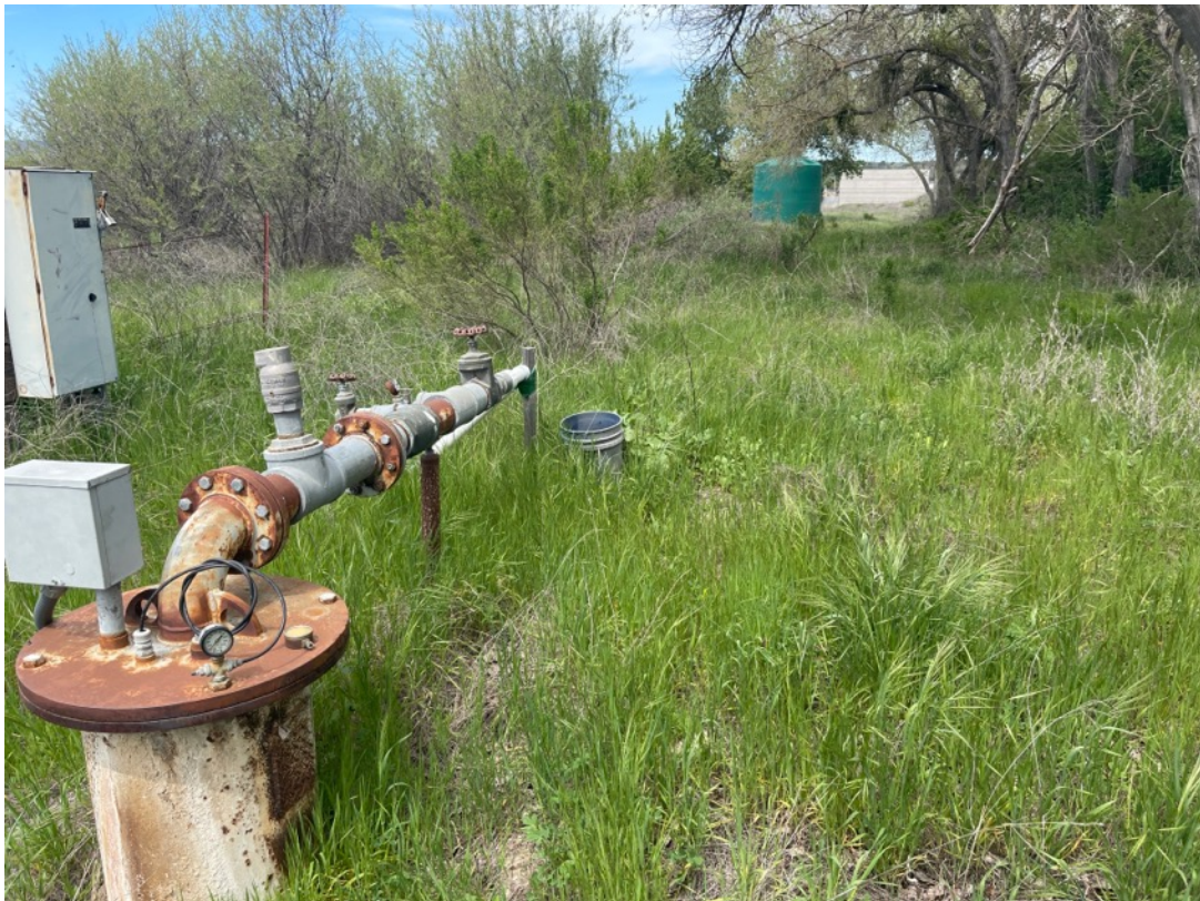
Photo 8. Southwest End of Narrow Extension, Facing Northeast.
