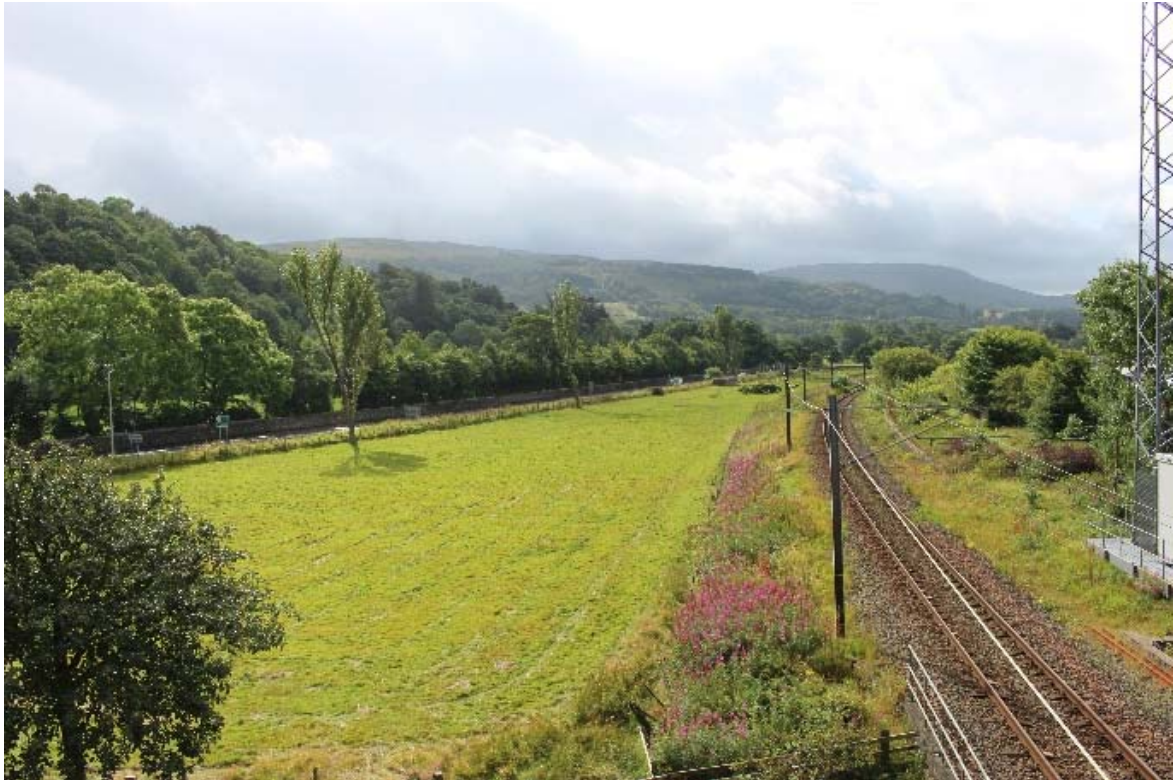
The narrow fields lying on the coastal edge between the railway line and the A78
