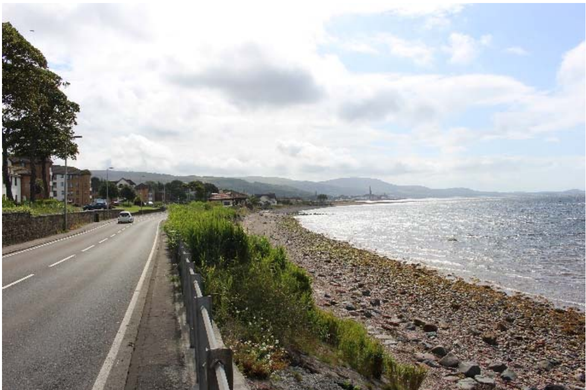
Linear development extends north along the raised beach platform far from the core of Largs
