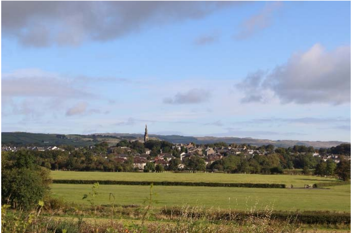
The attractive view of the historic core of Dalry from the south with the foreground of valley floor pastures forming AU A
