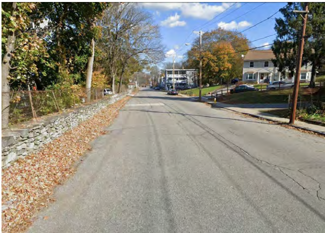
West Street has enough space to include a multi-use trail adjacent to the roadway.
