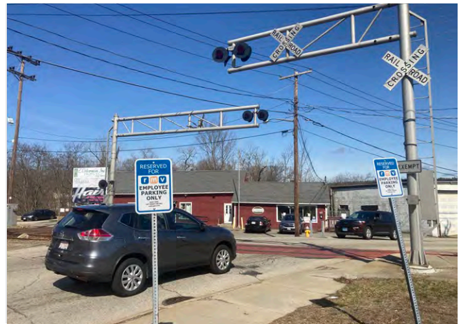
This section follows the rail-bed and there are several roadway crossings along this section. The crossings will need to have new safety features installed to increase pedestrian safety.
