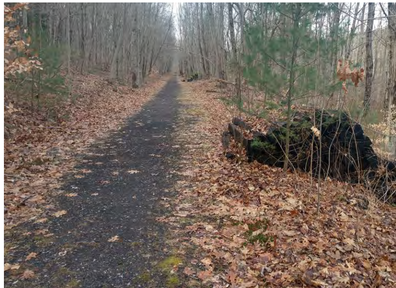
The abandoned railbed runs fairly consistently through the project area. Conditions vary as certain sections have been renovated over time to facilitate recreation in the area.
