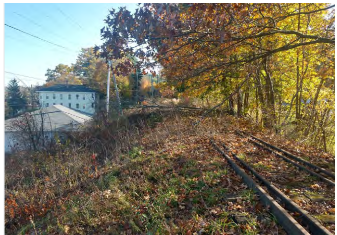
The elevated rail-bed will provide the proposed trail with good views.
