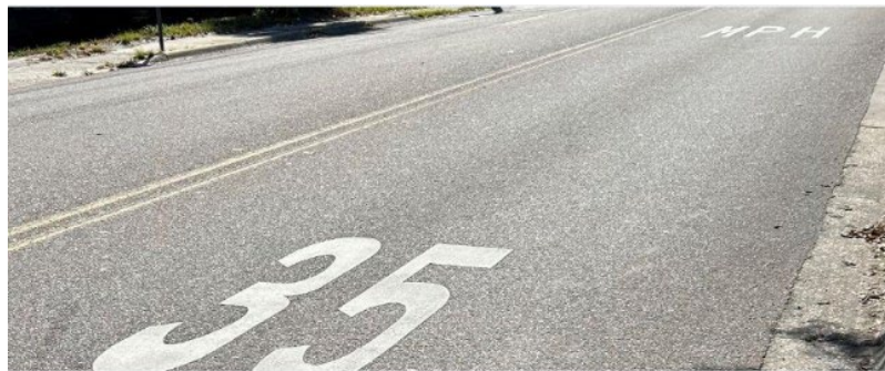
Enhance Pavement Markings at Neighborhood Gateways & Install Speed Limit Signage
