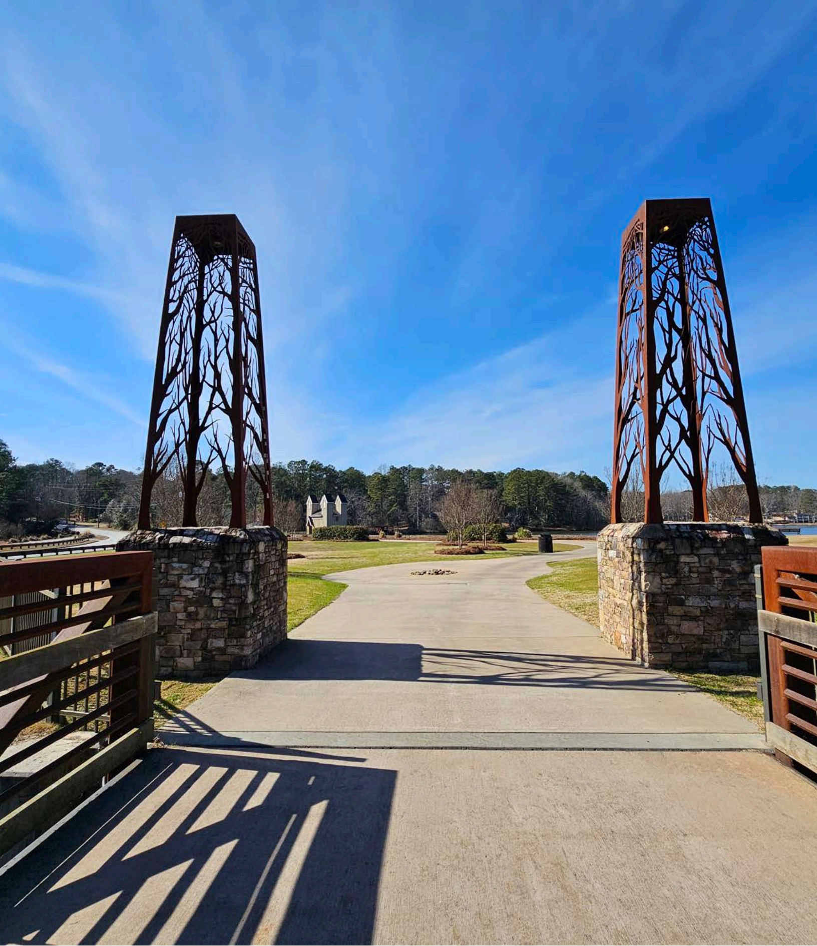
Lake Peachtree Dam & Spillway Park
