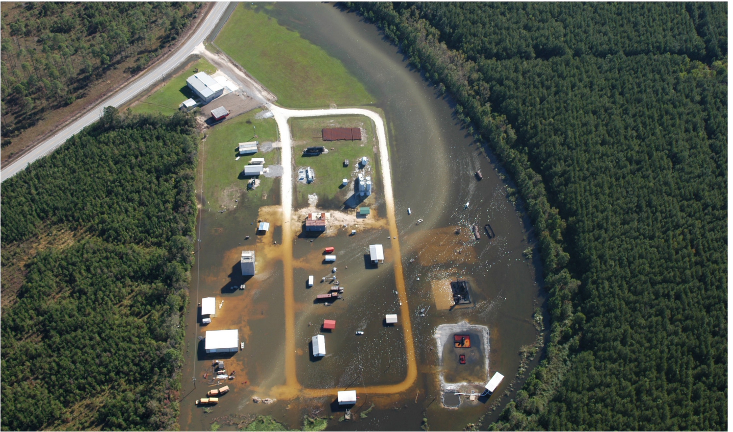
Figure 30: Flooding near Holbrook Park Road in northern Calcasieu Parish during the 2006 flood (CPPJ, 2006)
