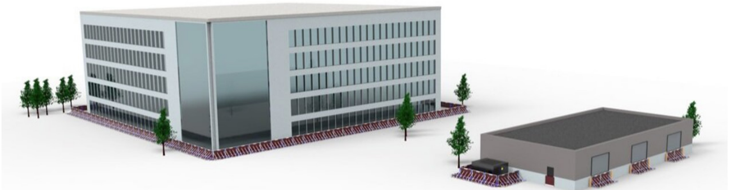
Figure 33: Floodproofing Around Commercial Structures
