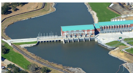
Image: Pump Station/Flood Gate Structure in New Orleans, LA
