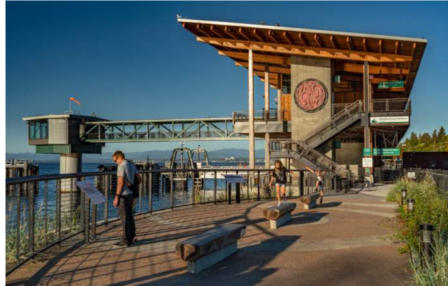
Mukilteo Ferry Terminal
