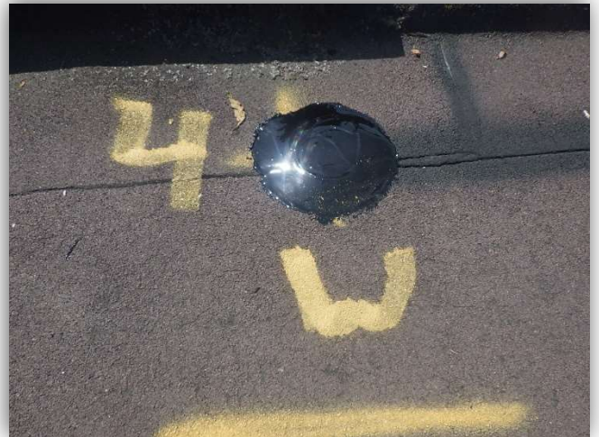
Probe #4 Roof Section 1.0 – Town Hall
