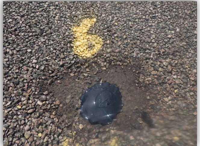
Probe #6 Roof Section 1.0 – Water Treatment Plant
