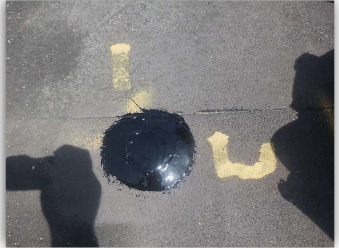
Probe #1 Roof Section 1.0 – Town Hall
