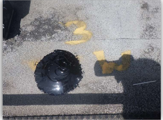
Probe #3 Roof Section 1.0 – Town Hall
