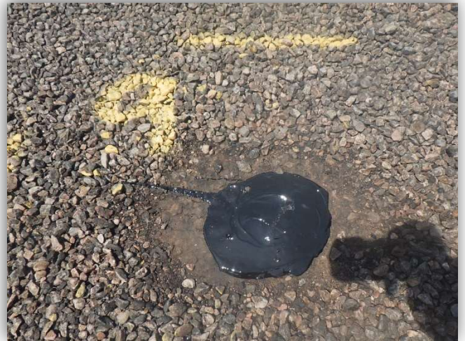
Probe #9 Roof Section 1.0 - Water Treatment Plant
