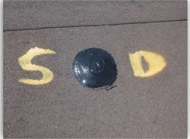
Probe #5 Roof Section 1.0 – Town Hall
