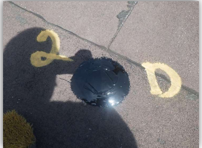
Probe #2 Roof Section 1.0 – Town Hall
