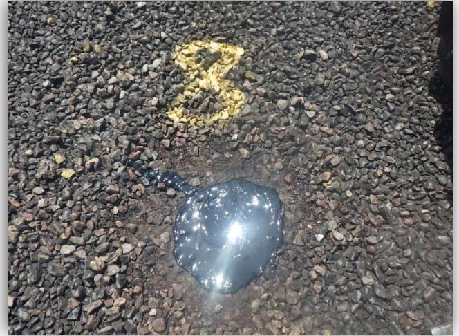
Probe #8 Roof Section 1.0 - Water Treatment Plant
