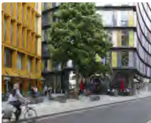
Two New Ludgate, Sauerbruch
