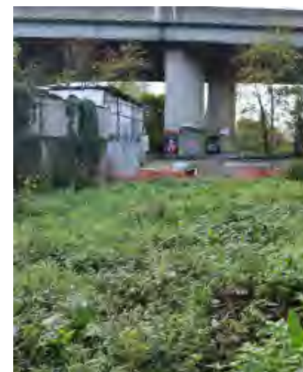
5. York Road (view looking west beneath north circular)
