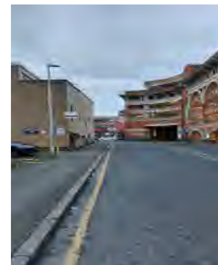
5. Exchange Ilford car park on Myrtle Road (looking south) Ilford OAPF 130
