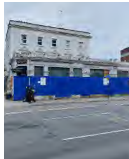
4. Former If Bar Building
