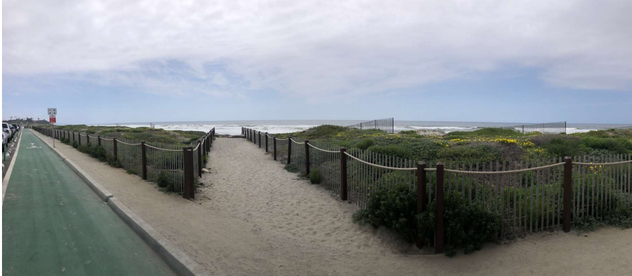
Cardiff State Beach Living Shoreline installed with a cycle track, decomposed granite path, and sand access pathways through the dune system
