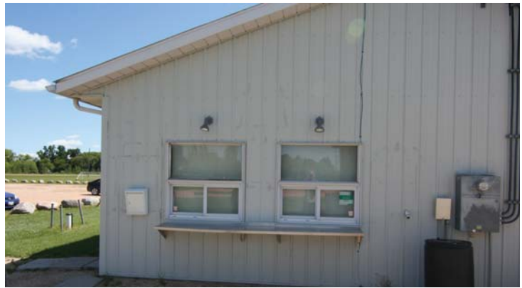
Exterior Service Windows from Kitchen
