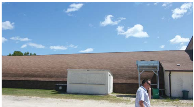
Exterior of Curling Rink Building and 1.5 Storey Building
