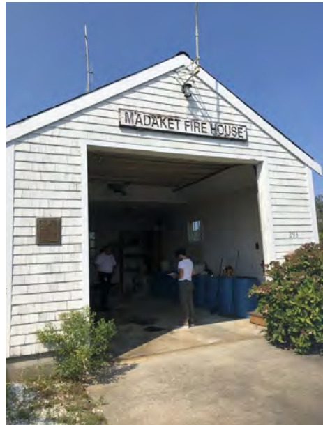
Storage barn – Madaket Fire House
