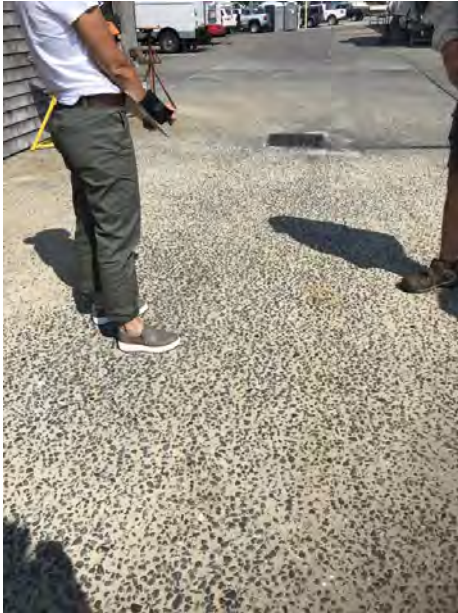
Catch basin outside of garage
