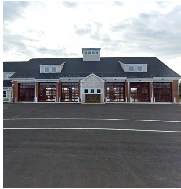
Front of building
