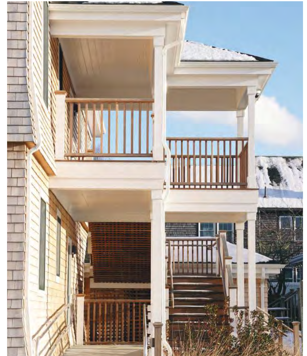
Seasonal workforce housing on Waitt Drive | December 2025
