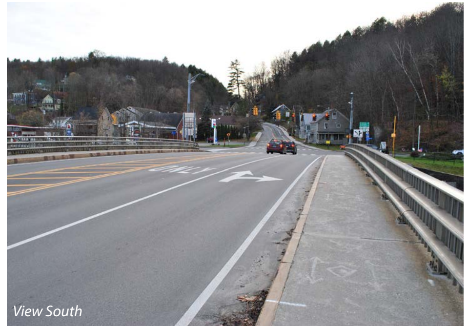
View South Figure 26: Main Street bridge
