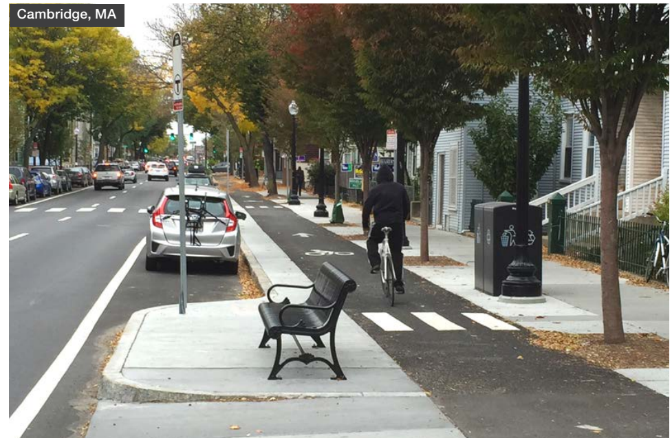
Figure 80: Bike lanes at sidewalk grade (Image courtesy of MassDOT)
