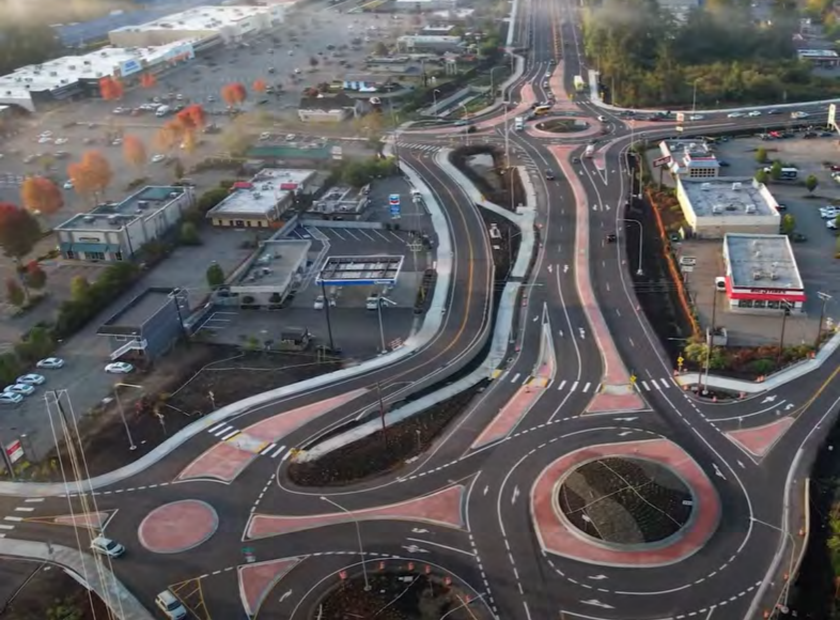
Four roundabouts were built near the intersection of State Routes 9 and 204 in Lake Stevens (Source: WSDOT)
