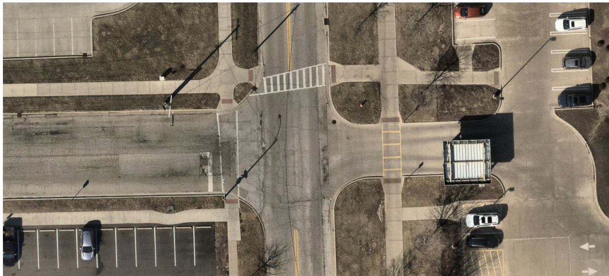
The intersection of University Street and Dale Street features pedestrian crossings that utilize three different pavement marking styles (Source: Nearmap).
