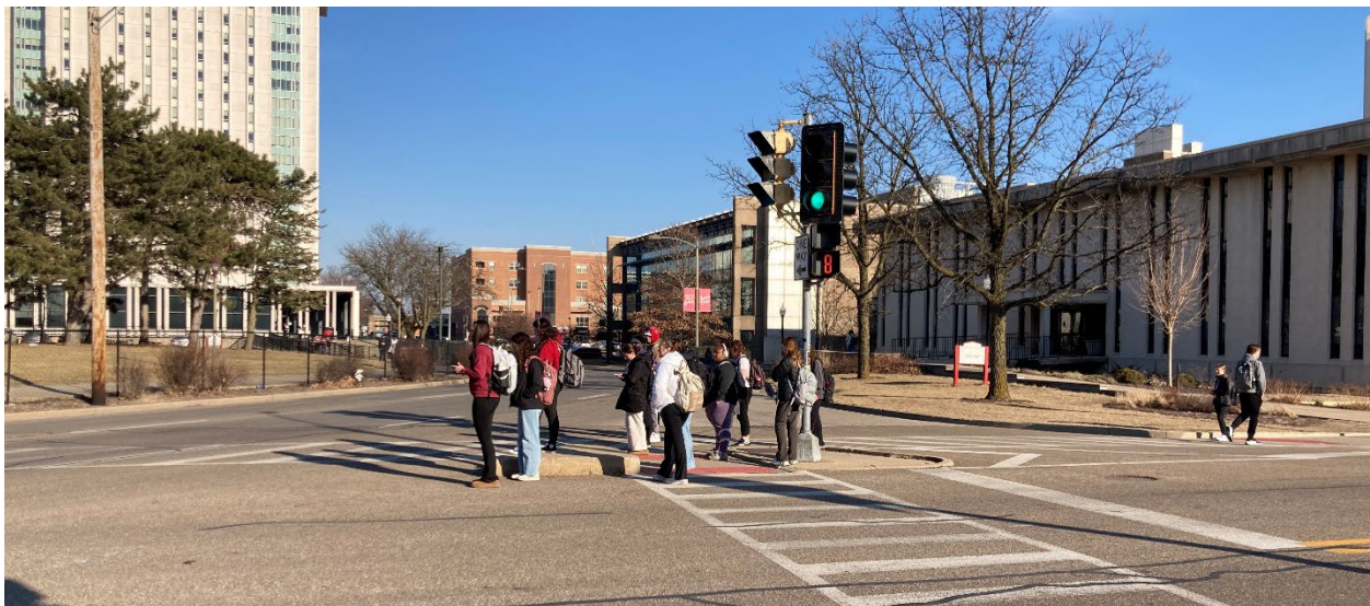
Pedestrians waiting to cross at the intersection of School Street and College Avenue. During peak hours, this triangular shaped island, or porkchop island, is not large enough to safely accommodate all users, requiring some people to stand in the street near passing vehicles.
