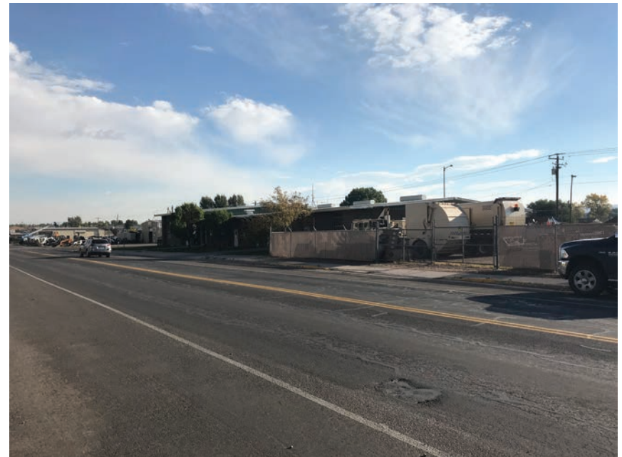
View of the Utility Building Looking North
