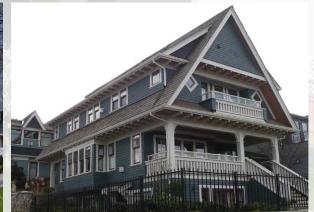
Kitsilano heritage house restoration
