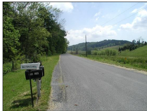
Looking north on State Route 252 in southern Augusta County.
