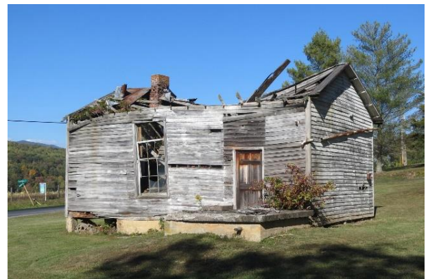
Estaline Schoolhouse, Virginia Department of Historic Resources
