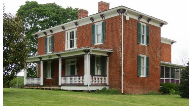
Harper House, Virginia Department of Historic Resources
