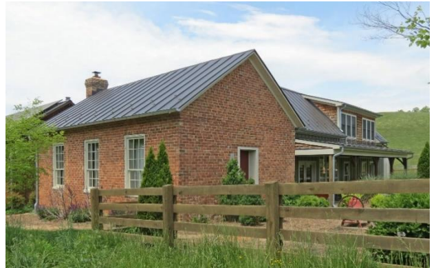
Glebe Schoolhouse, Virginia Department of Historic Resources
