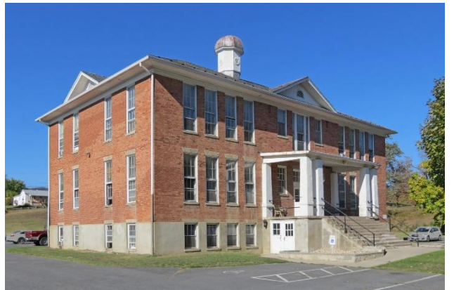
Craigsville School, Virginia Department of Historic Resources
