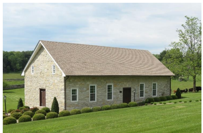
Old Providence Stone Church, Virginia Department of Historic Resources
