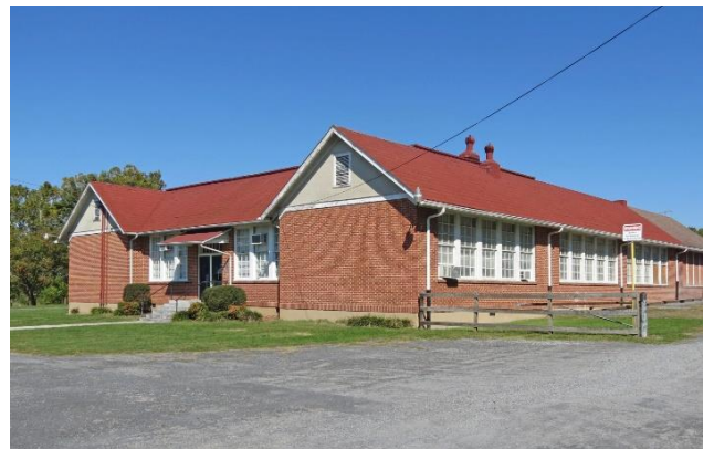
Crimora School, Virginia Department of Historic Resources
