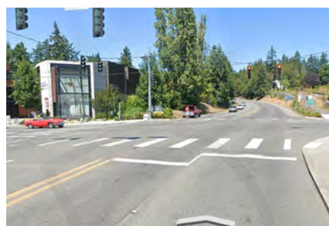
Distressed Pedestrian Crossing
