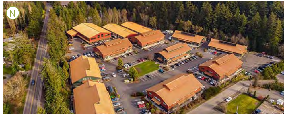
Copper Top development aerial view
