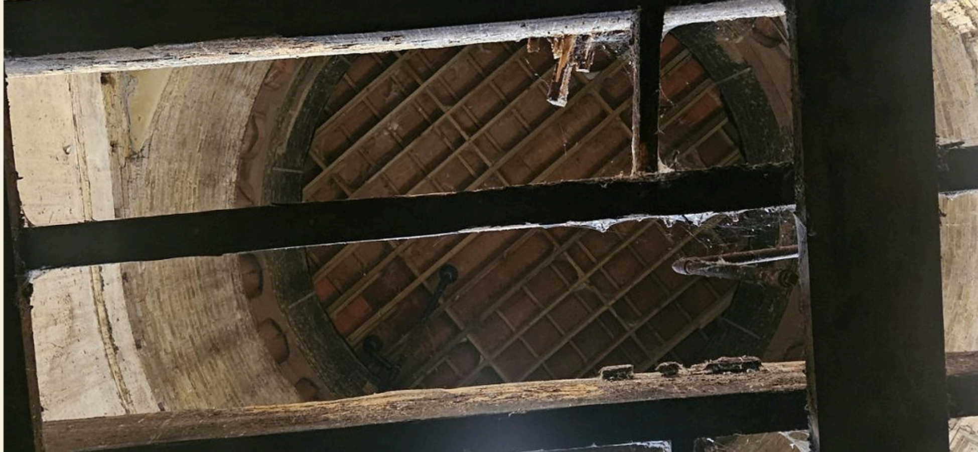
Inside the tower A timber stair climbing up inside the tower.
