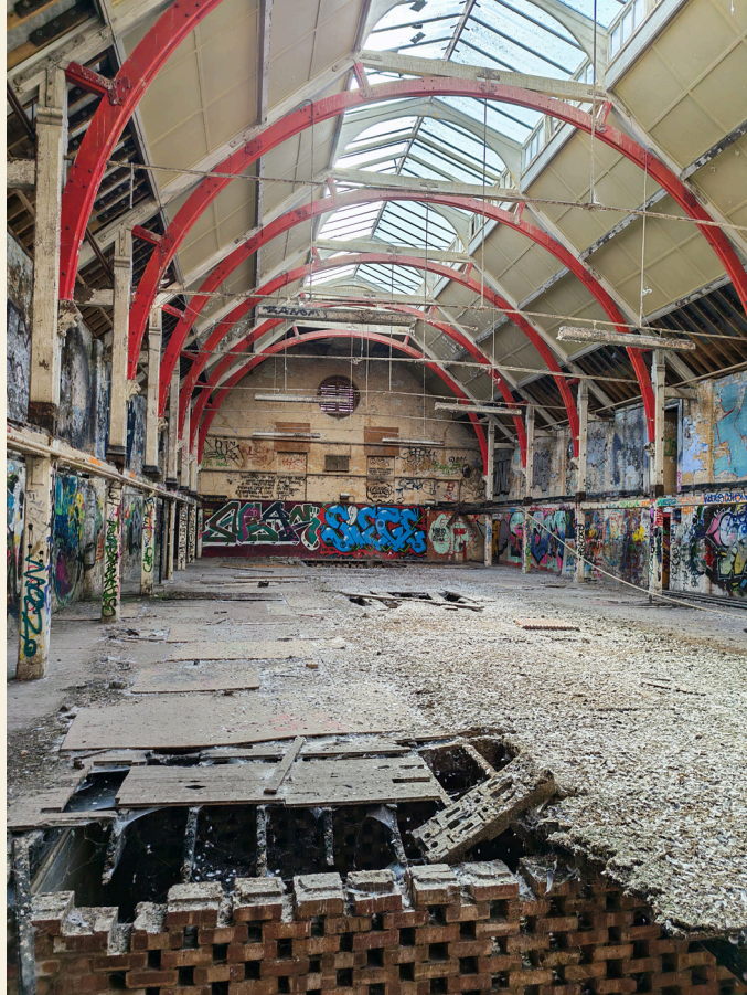
Arched roof + daylight Red steel ribs and a long glazed rooflight over the pool hall.
