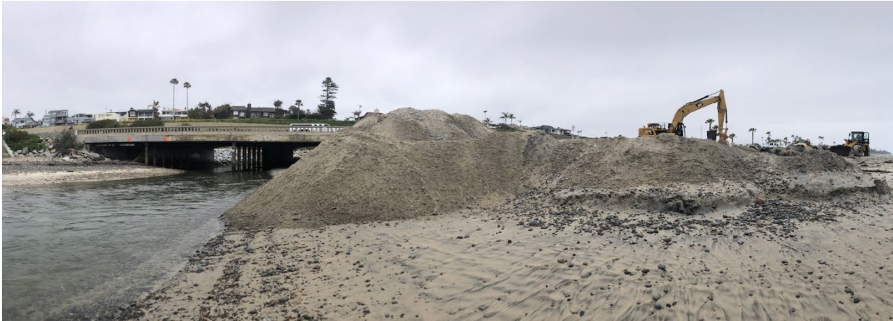
Dredging at Cardiff inlet at San Elijo Lagoon.
