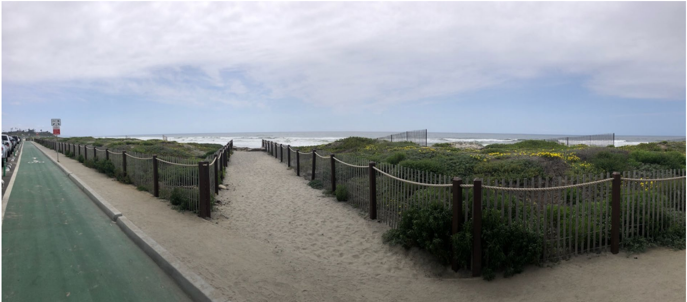
Cardiff State Beach Living Shoreline installed with cycle track, DG path, and access sand pathways through the dune system.
