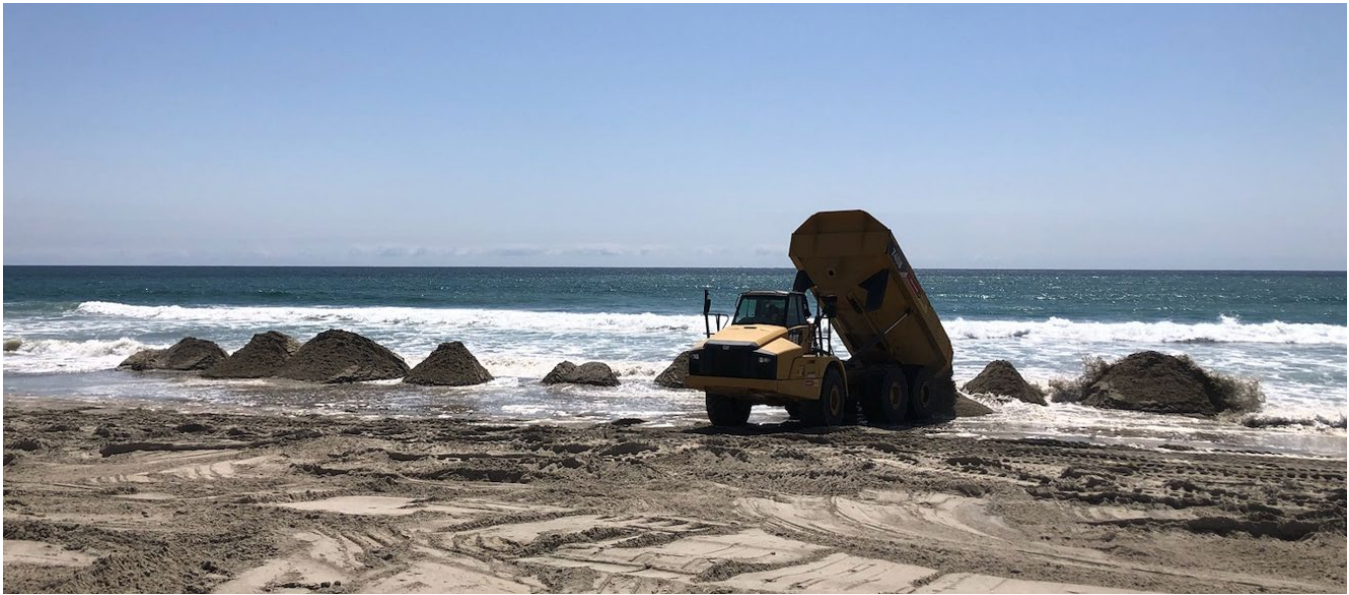
SCOUP placement at/along Cardiff State Beach within the intertidal zone for natural, longshore transport deposit.
