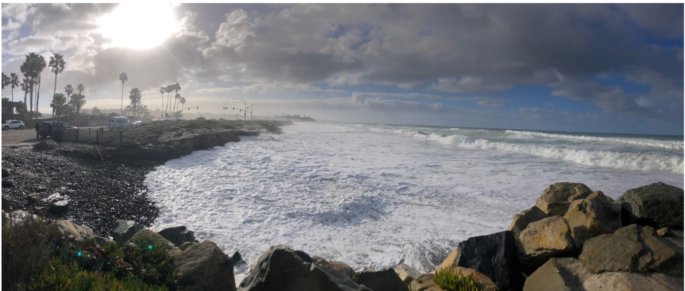
Storm surge onto the Cardiff State Beach Living Shoreline project during the 2024 El Nino storms.
