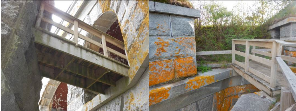
Photo 4.1 and Photo 4.2: Tier 2 (left) and Barbette Tier (right) bridges
