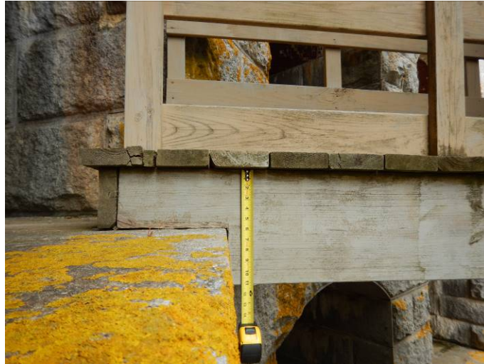
Photo 4.7 Bearing end of Tier 2 Bridge at Casemate 246.
