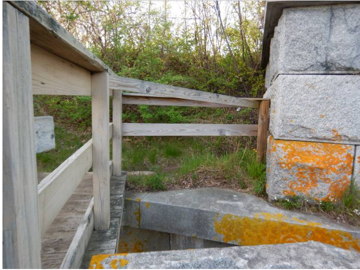
Bridge and Barbette Tier Railings
