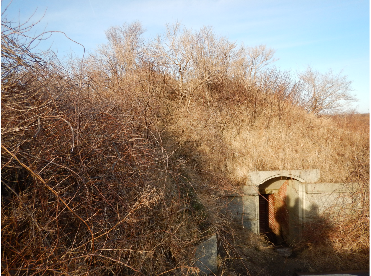
Above: Barbette Tier, Built-up berms (parados) over passageways to Barbette Tier powder magazines. Below: Scrub foliage reduces and obscures the visibility of parados (left), an important historical feature of the fort. More visible contours are viewed from parade ground (right)
