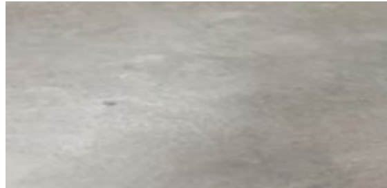
POLISHED CONCRETE FLOOR
