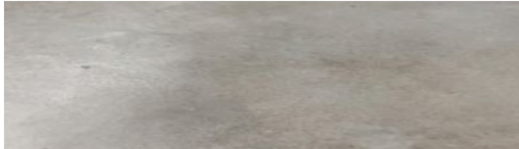
POLISHED CONCRETE FLOOR
