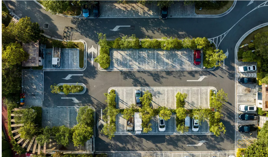
Parking Lot Improvement, Lincoln, NE
