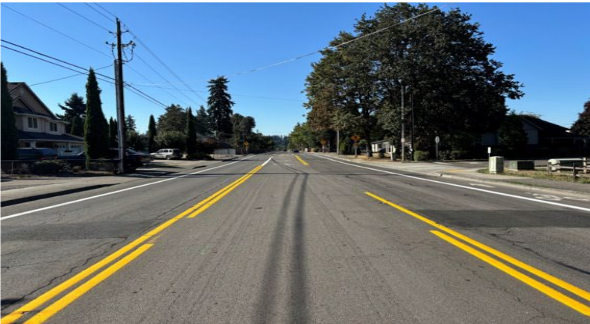
Figure 10: At the intersection of Northeast 86th Avenue and Northeast 33rd Street, which accesses Ogden Elementary school, there are single lanes of traffic in each direction plus continuous center turn lane. There are sidewalks and striped bike lanes on both sides of Northeast 86th Avenue.
