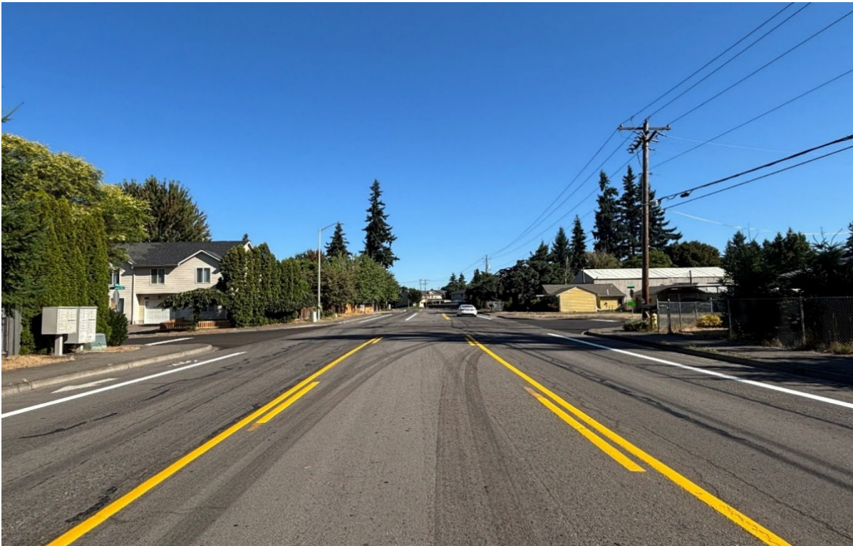
Figure 11: At the intersection of Northeast 86th Avenue and Northeast 36th Street there are single lanes of traffic in each direction plus continuous center turn lane. There are sidewalks and striped bike lanes on both sides of Northeast 86th Avenue.
