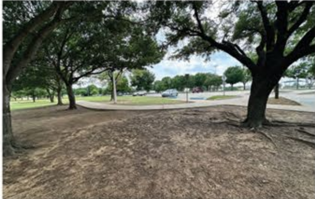
This image shows some erosion on the site due to the slope and the unmitigated water flow.
