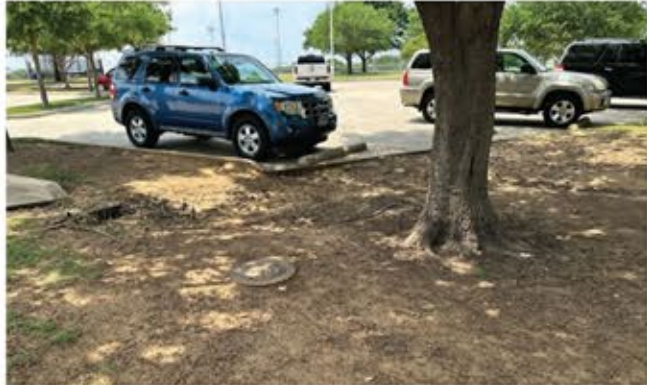
This image shows some of the major erosion directly off of the parking lot.
