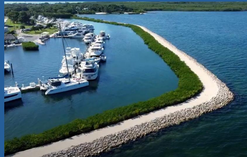
Founders Park Breakwater | Islamorada, FL
