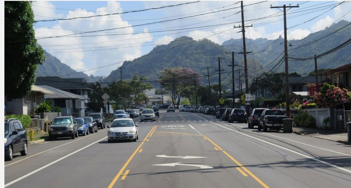
Lane Repurposing / Center Turn Lane
