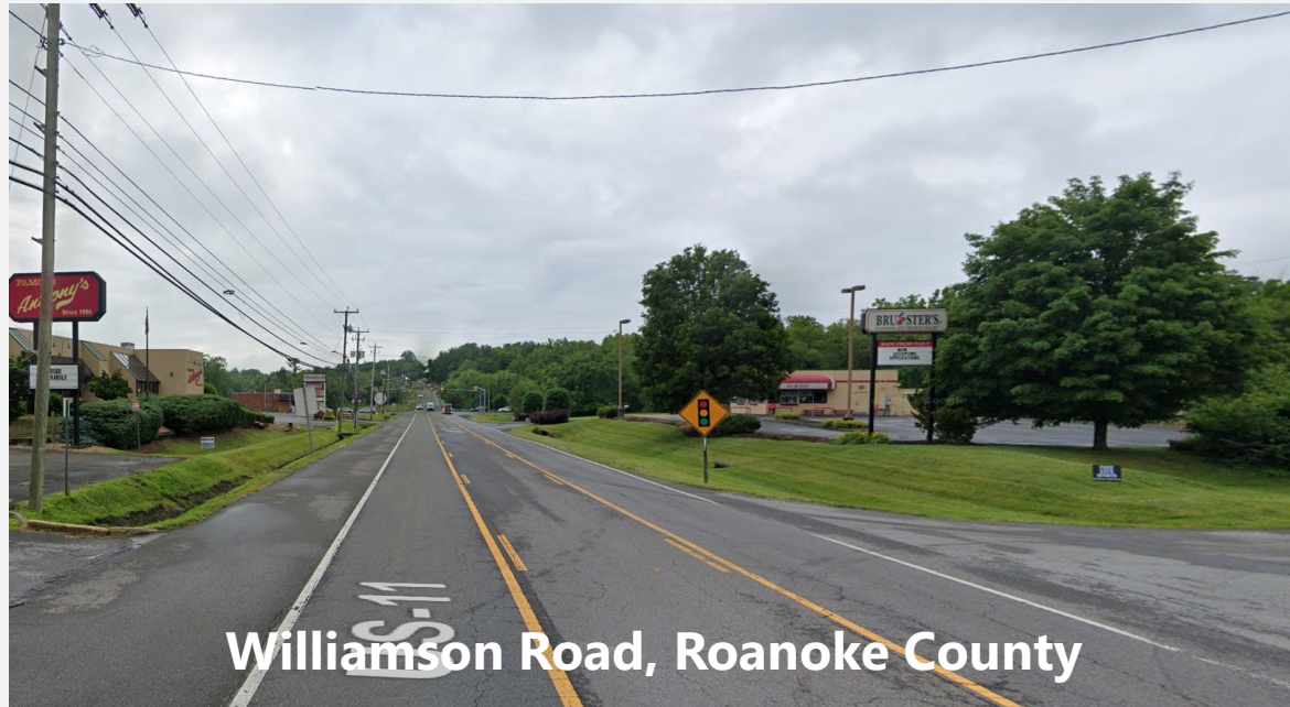
Two-way Left-Turn Lane
