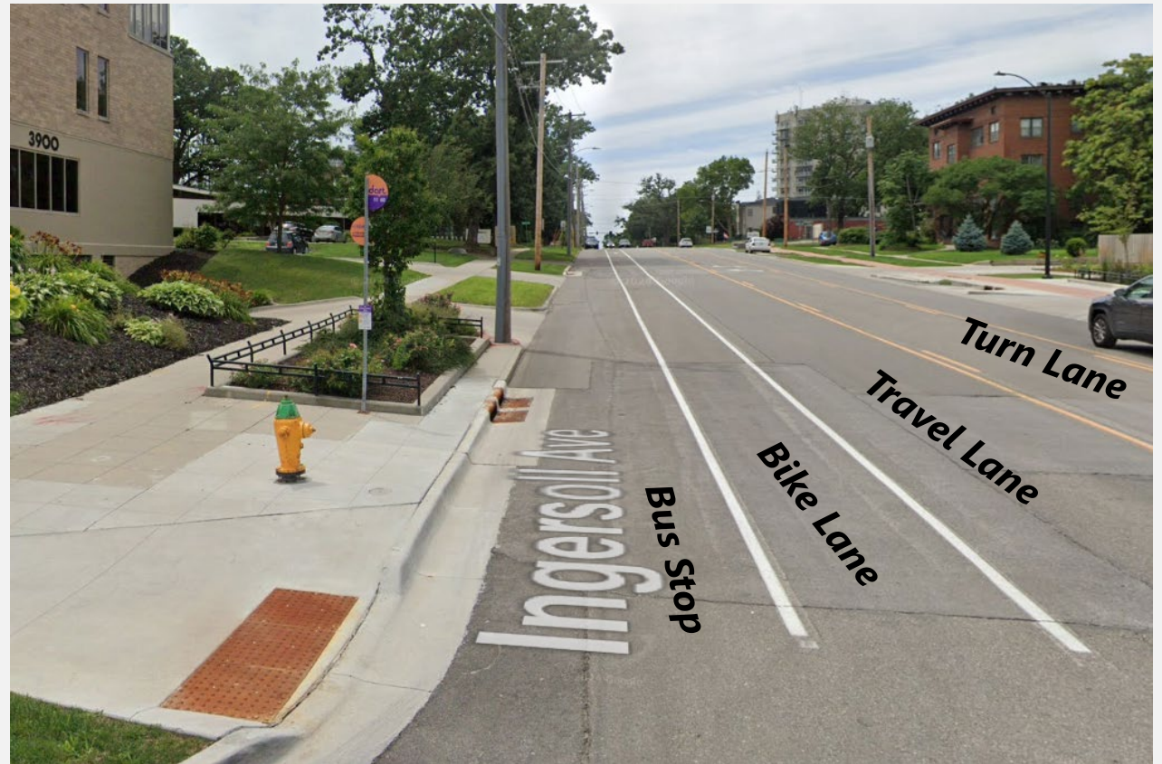
Center Turn Lane with Bike Lane & Bus Stop Pull-off
