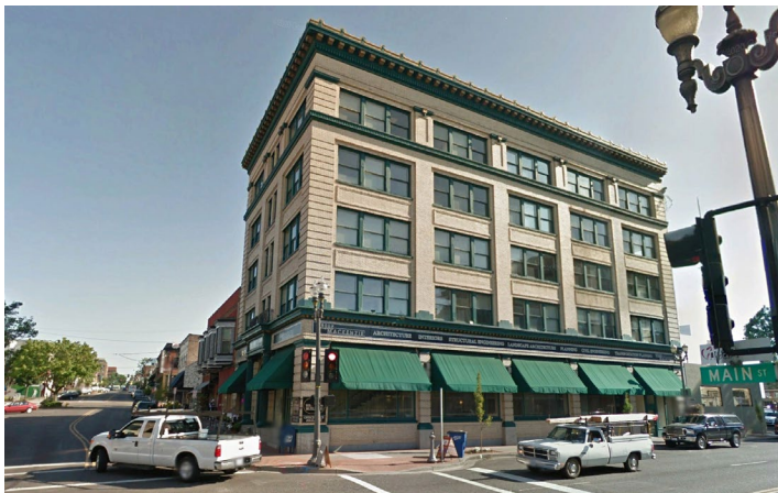
Example of the use of cornice lines at the base and top of the building to define the three portions of the facade.
