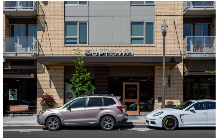
Example of a prominent and easily identifiable primary entrance.
