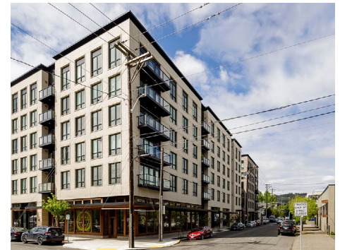
Example of building with multiple modulations that extend from the ground floor through the roof plane.
