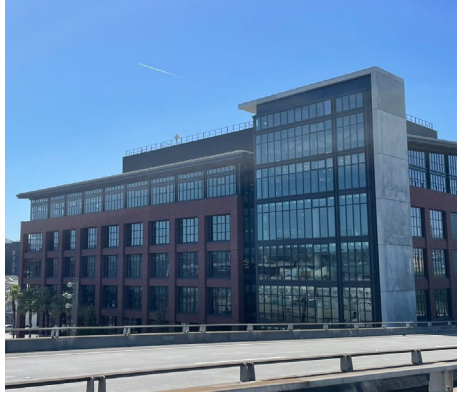
Example of a building with glass curtain walls that do not exceed 50% of any single facade.
