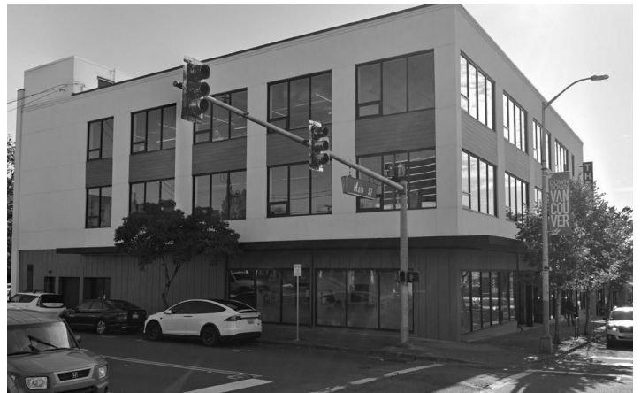
DON'T Stucco should be limited. Materials in the Heritage District should complement existing buildings and reinforce the character of the area.
