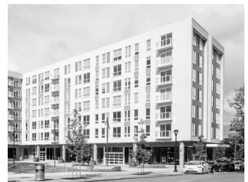
DON'T: Create flat facades with only balcony projections and no facade modulation that result in an overly flat facade appearance.
