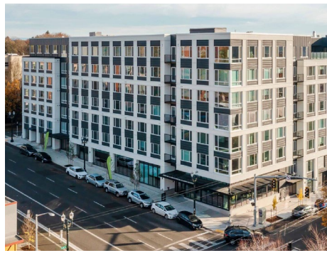
Example with two modulations that break the facade into three distinct massing elements. The breaks are emphasized with a change in color and material. Modulation and articulation of the ground floor complement and align with upper floors.
