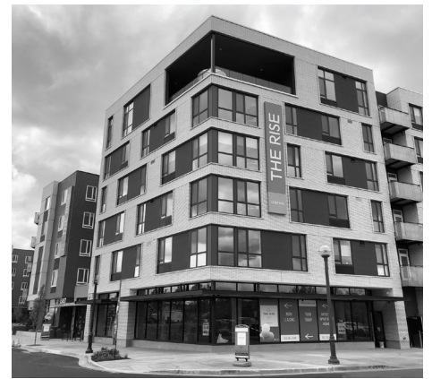
DON'T Design over dominating building signage that does not complement facade composition and materiality.
