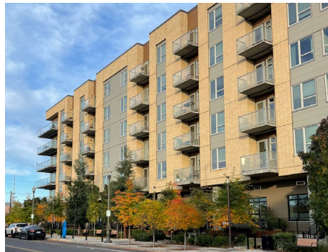
Example of building with multiple modulation recesses with balcony projections. Modulations begin at the second floor.
