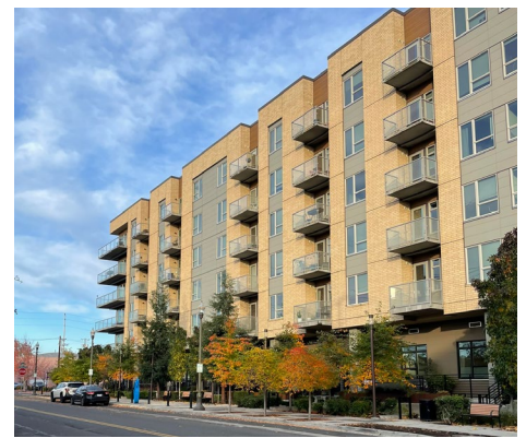
Example of facade with multiple modulいたions with an approximate depth of 3 feet.
