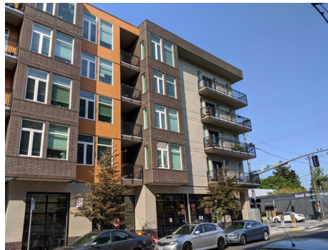
Example of facade modulation extending through the roof plane creates distinct upper floor massing elements.
