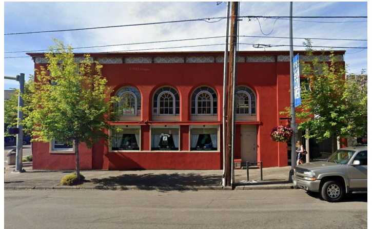
Example of a building with well articulated ornamentation, artistic fenestration pattern and cornice.
