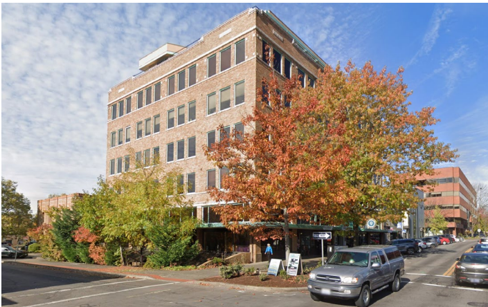
DO Use materiality and fenestration pattern that are consistent with the character and identity of the Heritage District.
