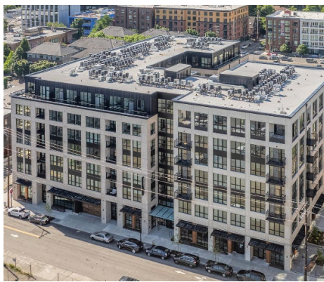
Example of facade with single major break.
