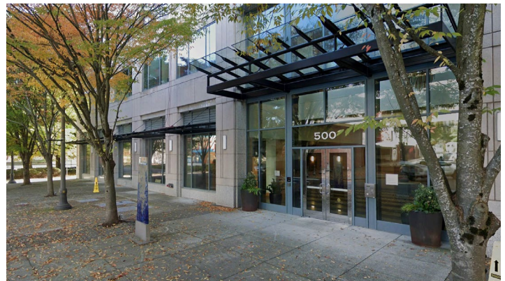
Example of a primary building entrance awning that is higher than the adjacent awning.
