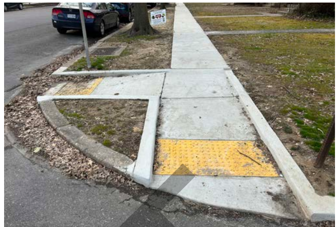
New curb ramp
