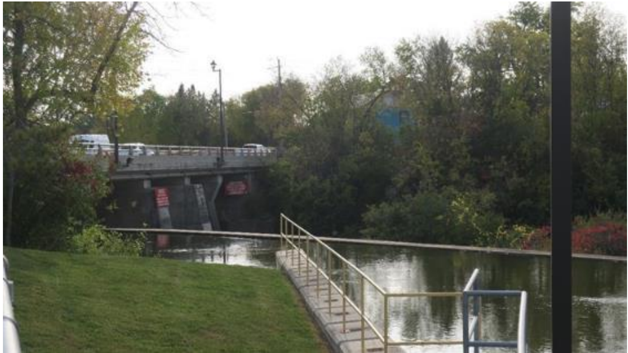
Photo 7: Existing Raglan Street Bridge crossing Bonnechere River
