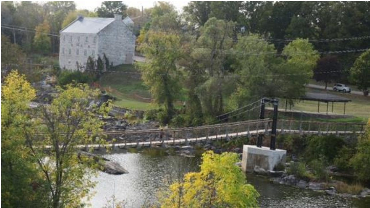
Photo 6: Existing Pedestrian Bridge across Bonnechere River
