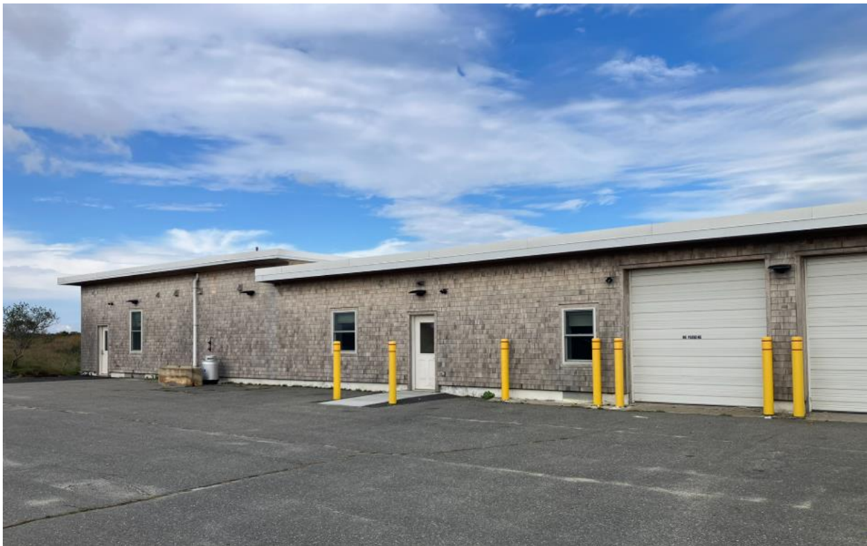
Figure 5- Women's Dormitory exterior improvements
