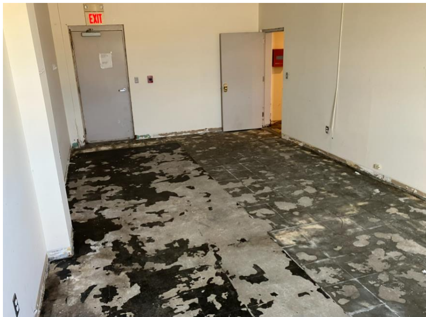
Figure 4- Asbestos floor tiles removed
