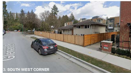
3. SOUTH WEST CORNER
