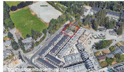
5. SOUTH LOOKING NORTH (AERIAL)
