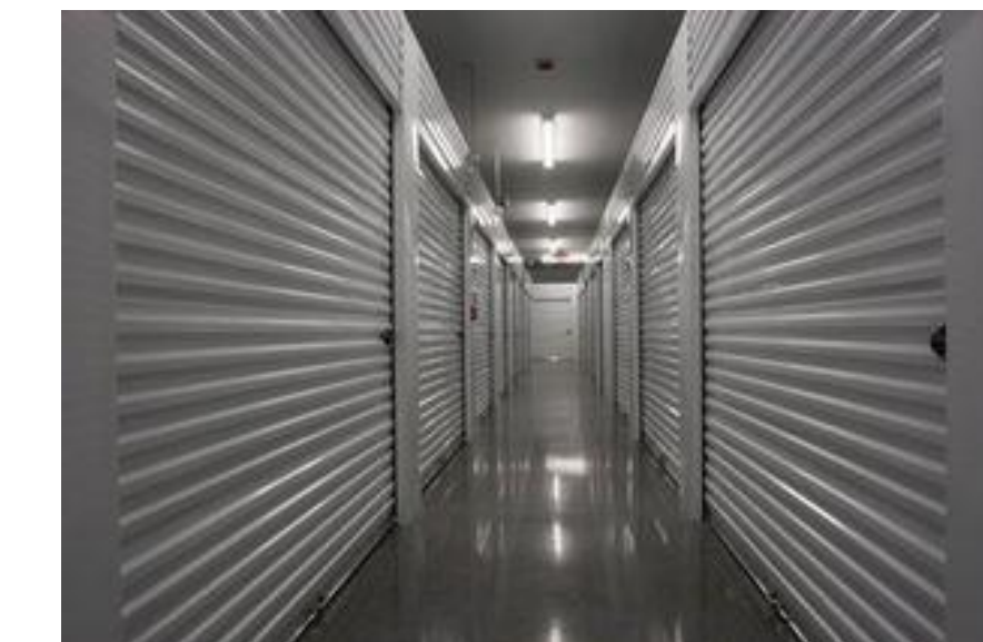
Source: A Friendly Storage, www.afriendlystorage.com
