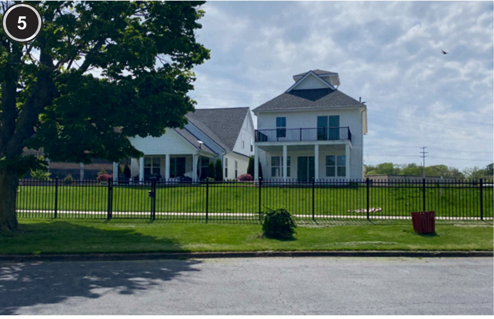
5 ORNAMENTAL PERIMETER FENCE. FENCING IS ATTRACTIVE AND IN GOOD CONDITION
