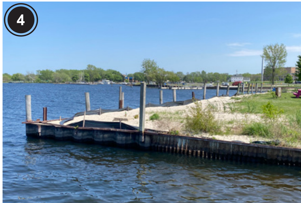
4 EXISTING SHEET PILE WALL
