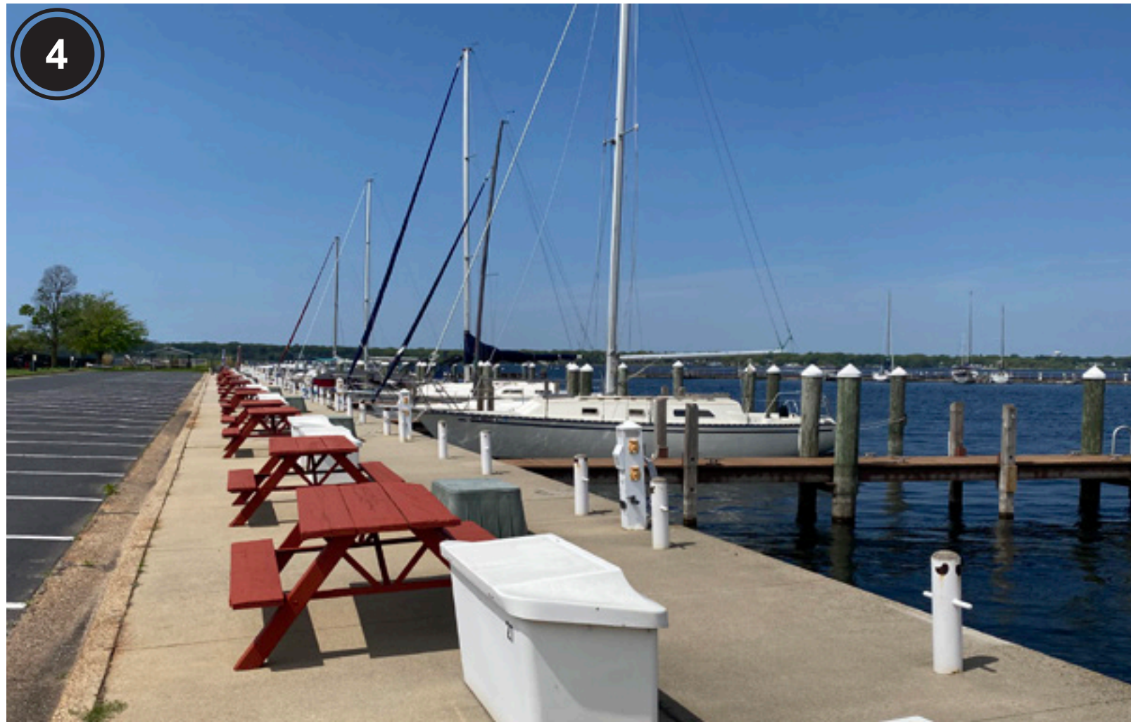
4 TYPICAL DOCK SETUP. NOTE THAT THERE IS NO ACCESSIBLE ACCESS TO THE DOCKS
