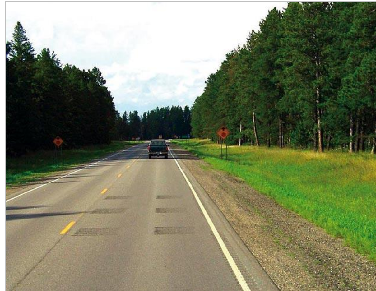
Source: FHWA / MnDOT
