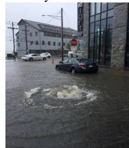
Photo: Flooding at the Maple Street/Commercial Street Intersection on 8/18/2023
