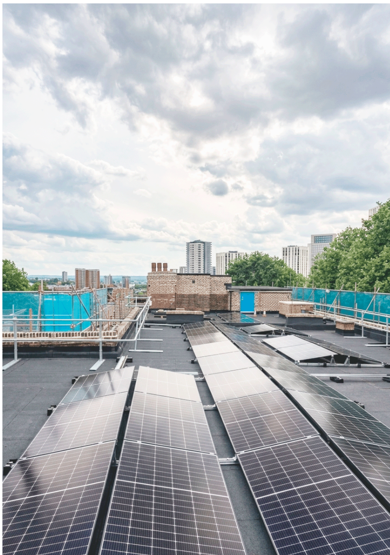
Solar panels were installed on The Hermitage in 2024.
