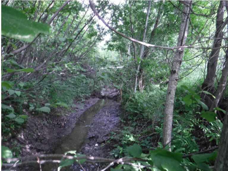
Photo 8 – Site Conditions of Pleasant View Municipal Drain Along Southeastern Property Line. View Looking Northwest. Photo Taken June 17 2022.
