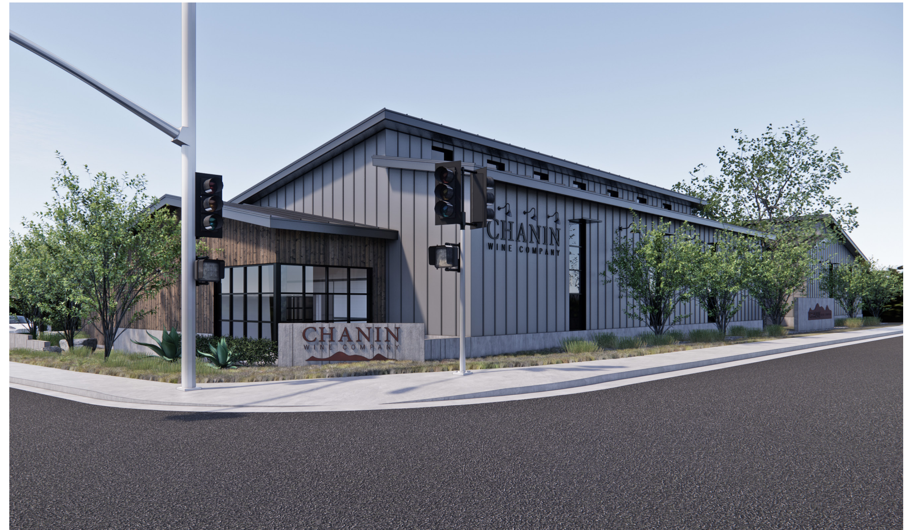
CORNER OF INDUSTRIAL WAY AND HIGHWAY 246
