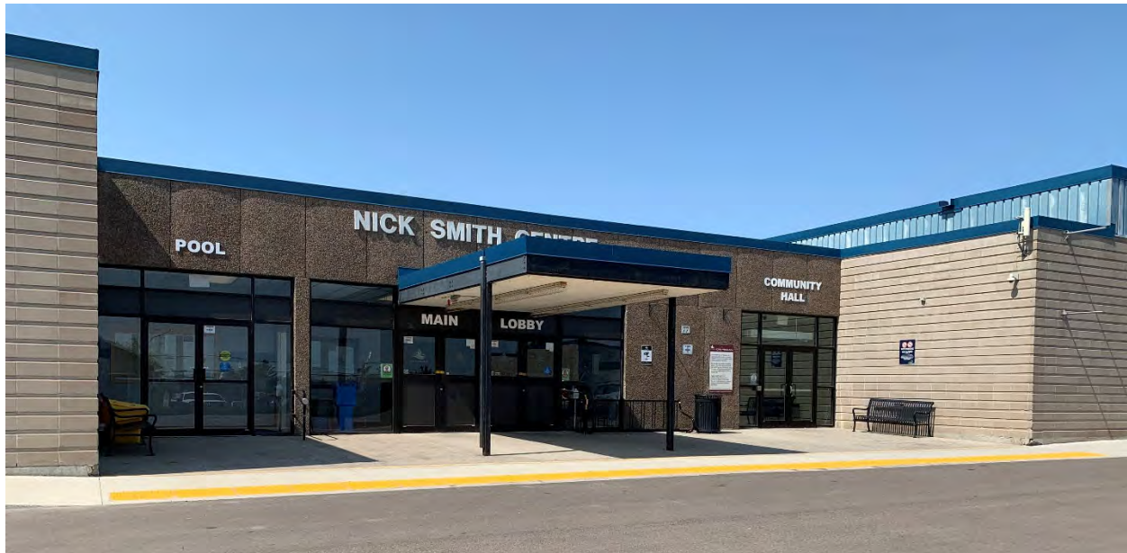
Figure 18 – Nick Smith Centre Entrance
