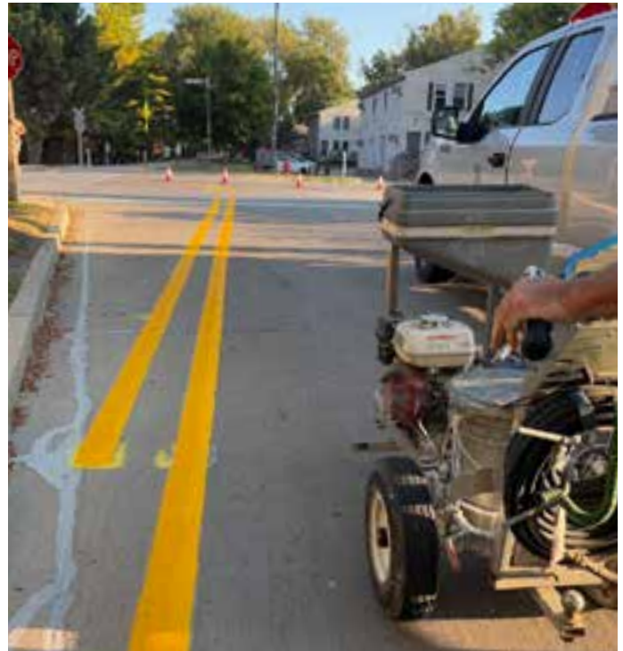
Department of Public Works staff install striping on Constitution Boulevard.
