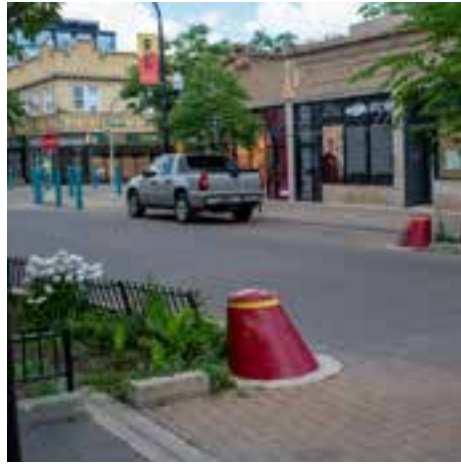
Shared street on Argyle Street in Chicago, Illinois
