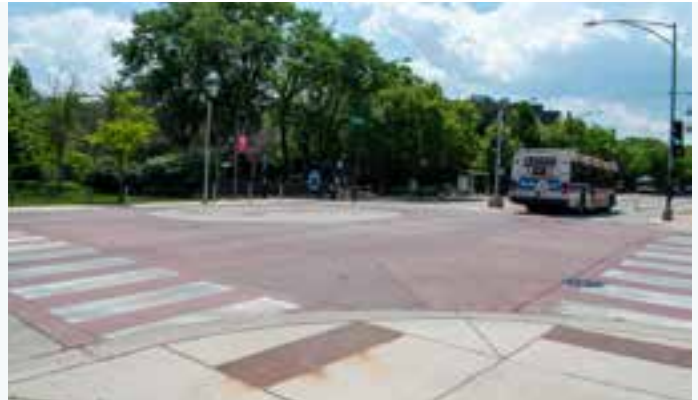
Colored concrete at the University of Illinois at Chicago
