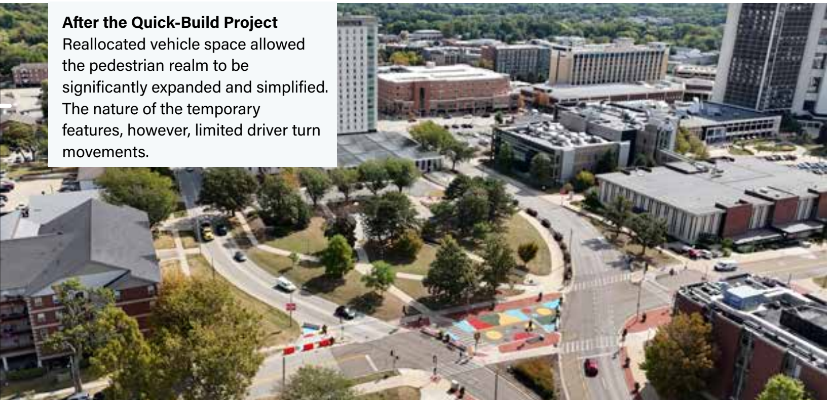
Oblique aerial image of School Street between Mulberry Street and College Avenue after quick-build project installation, facing southeast.
