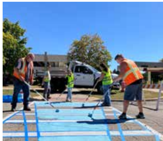
Project team members paint a crosswalk
