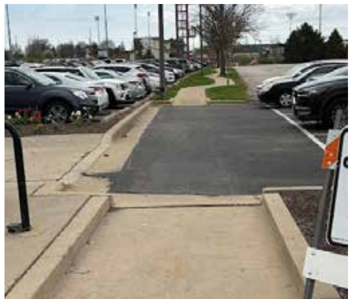
Constitution Trail east of Tri-Towers between G82 and S81 parking lots
