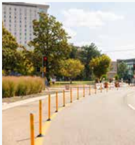
Yellow plastic bollards installed in the existing hatched area on College Avenue approaching School Street.
