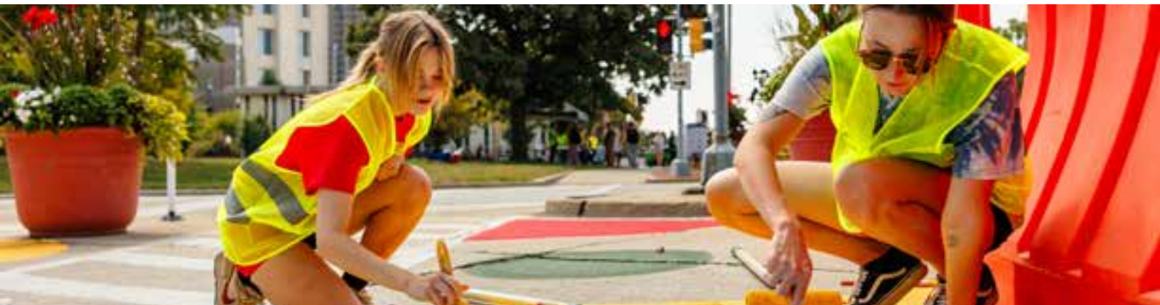
Students painting the closed turn lane on Mulberry Street at School Street.
