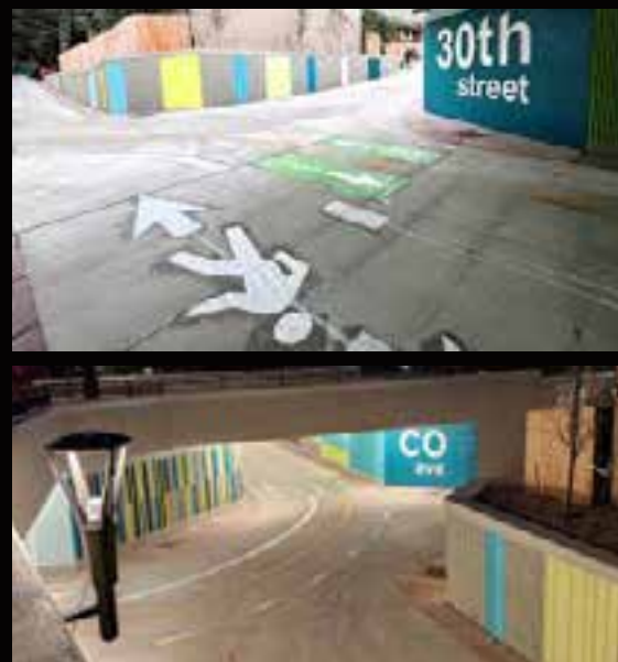
30th Street and Colorado Avenue underpasses (Photo/City of Boulder, Colorado)
