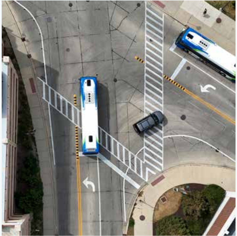
Aerial view of Fell Avenue at Beaufort Street with left turn hardened centerlines, and reduced crossing distances through white paint and flexible posts. Two buses approach the intersection and a vehicle turns right.
