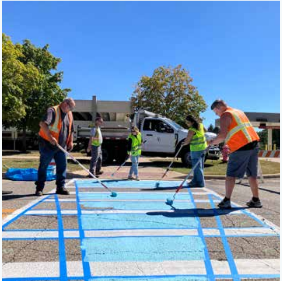
Project team members paint a crosswalk with blue paint on University Street.
