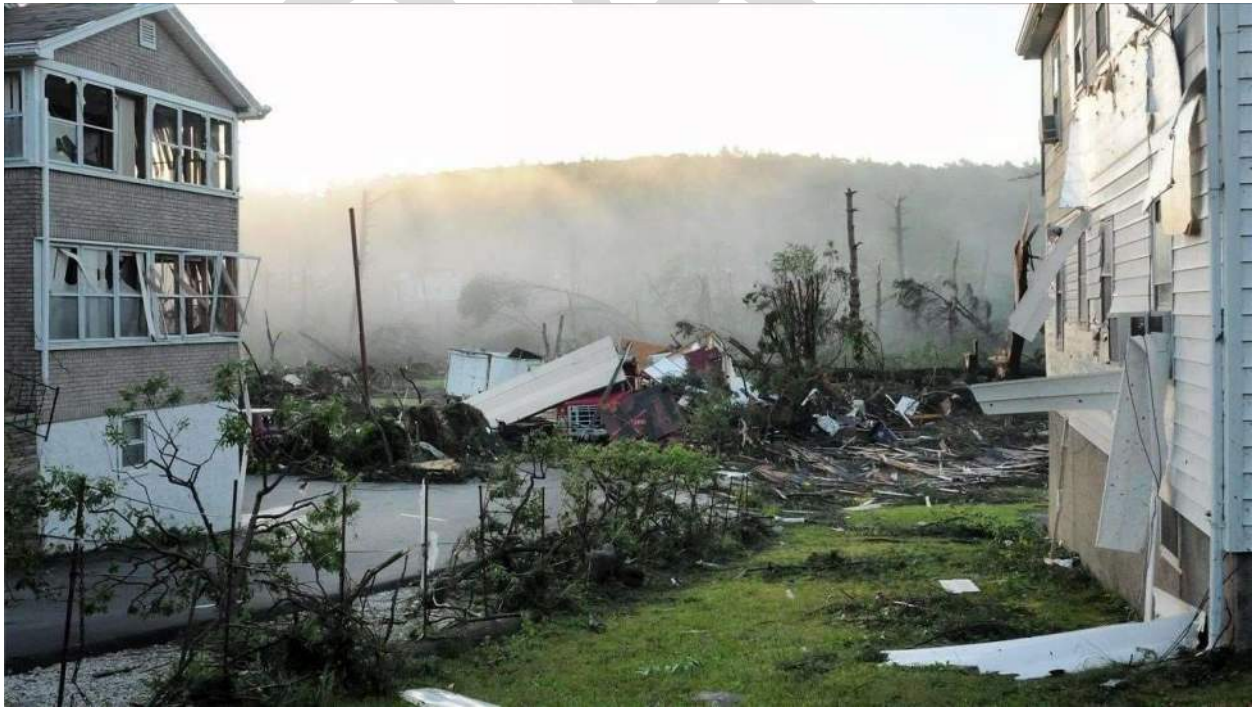
Tornado Damage, Photo courtesy of Fire Chief Paul Normandin
