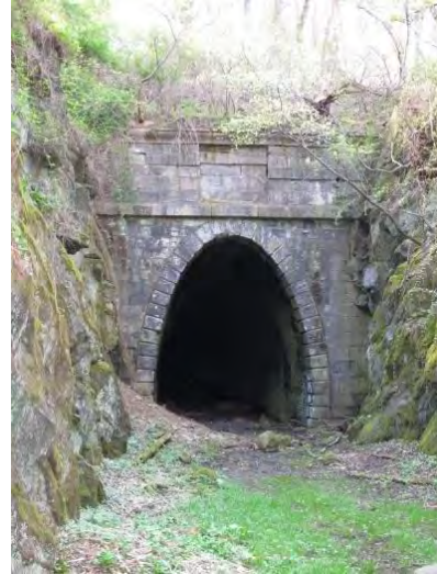
Blue Ridge Tunnel, Virginia Department of Historic Resources
