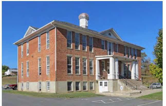
Craigsville School, Virginia Department of Historic Resources
