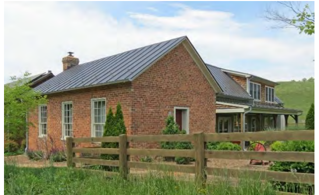
Glebe Schoolhouse, Virginia Department of Historic Resources
