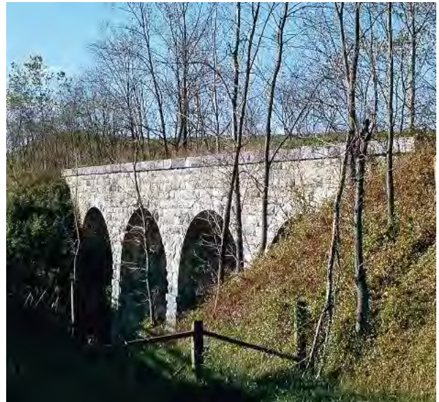
Valley Railroad Stone Bridge, Virginia Department of Historic Resources
