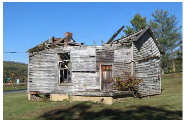
Estaline Schoolhouse, Virginia Department of Historic Resources
