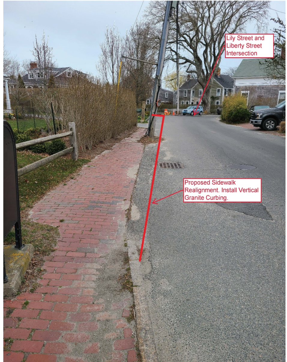
FIGURE 3 - LIBERTY STREET SIDEWALK REALIGNMENT
